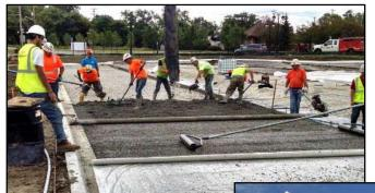
At left, workers from contractor Fessler & Bowman place pervious concrete at the Red Fox Outfitters parking lot. Construction was managed by Rhoads & Johnson. Below is the Red Fox Outfitters building.
