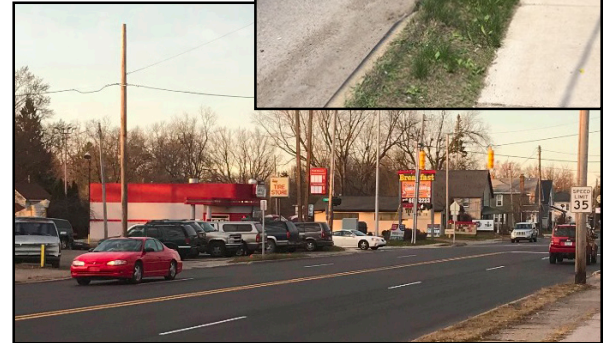
A before and after view of approximately the same stretch of Saginaw street.
