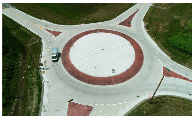
Dort Highway Extension Roundabout
