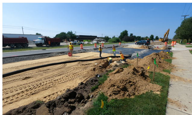
Crews working on new drainage
