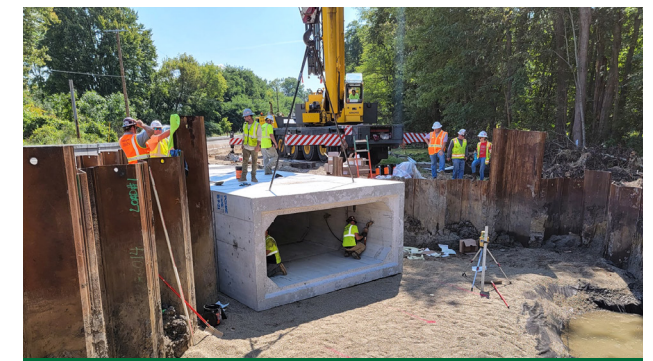
Culvert being lowered into place
