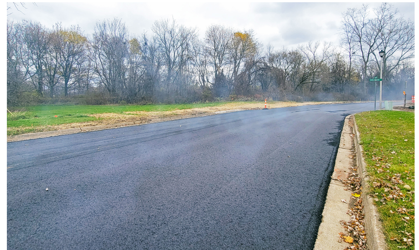
Vinewood Street Resurfacing
