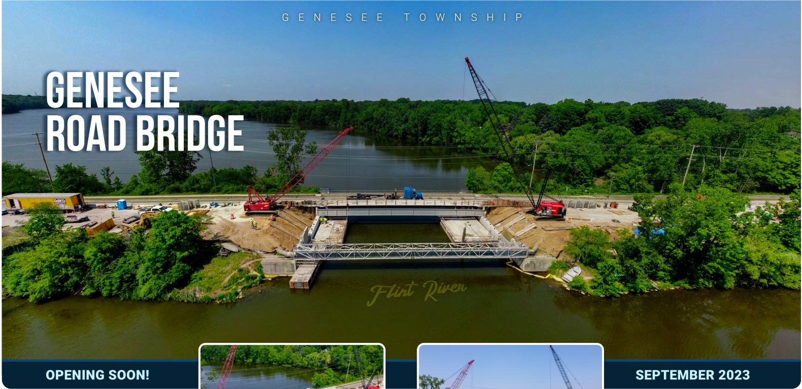
The new steel girders have been placed on the east half of the bridge and concrete work is ongoing. Genesee Road will be maintained in its current configuration through the rest of Stage 1, then traffic will be shifted onto the new half of the bridge for Stage 2. The project is on schedule to be completely open to traffic September 15,
